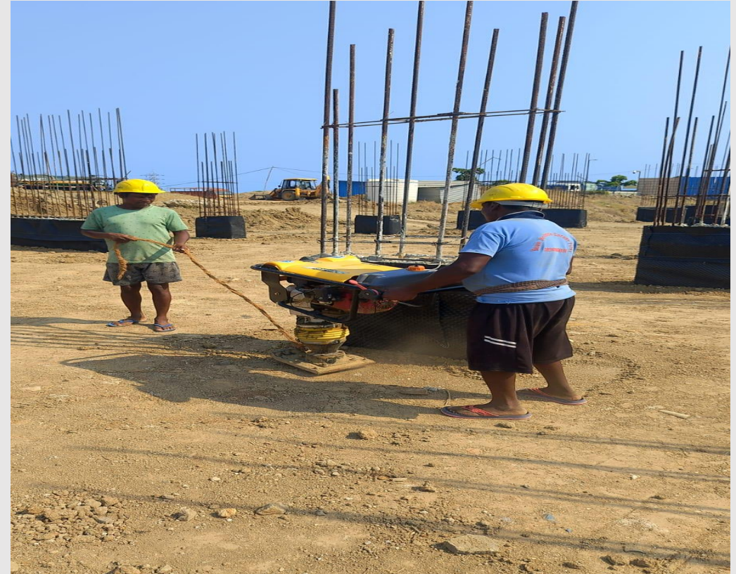
Plate compaction work in progress
