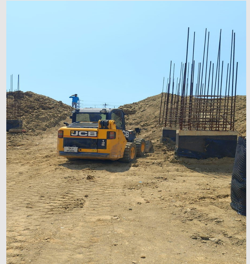
Earth Leveling work in progress
