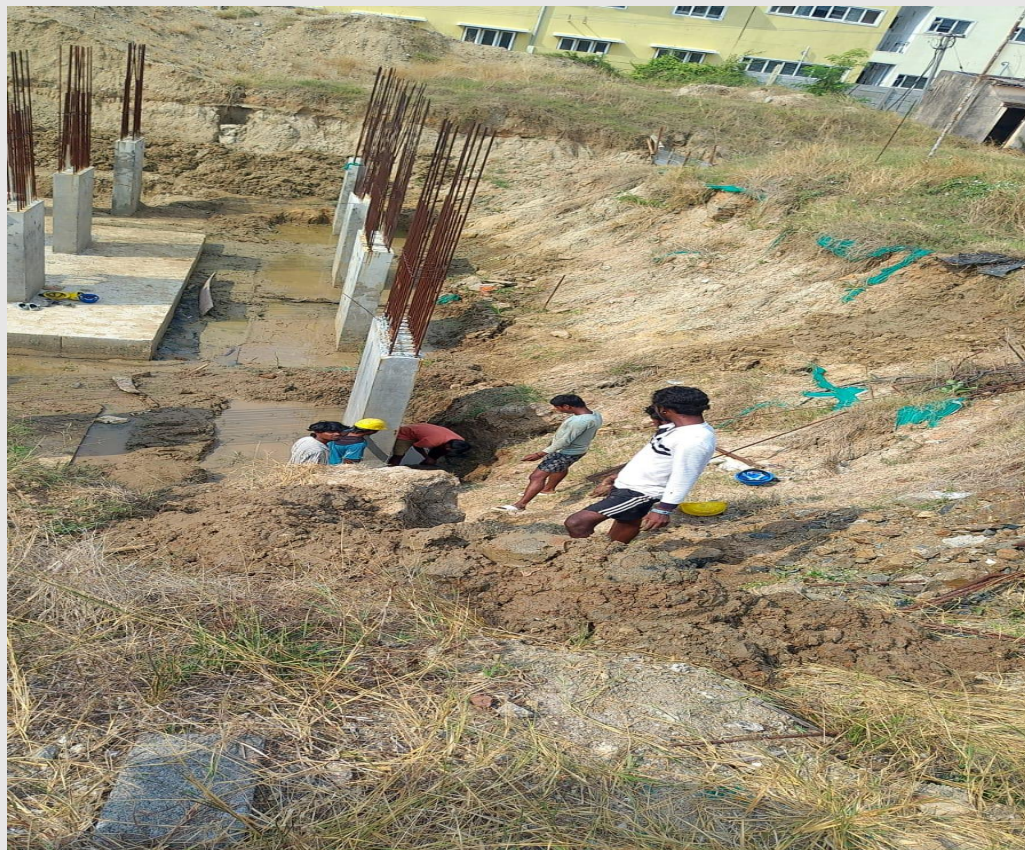
Slush cleaning work in progress
