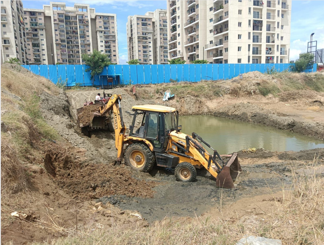
Slush cleaning and dewatering in progress
