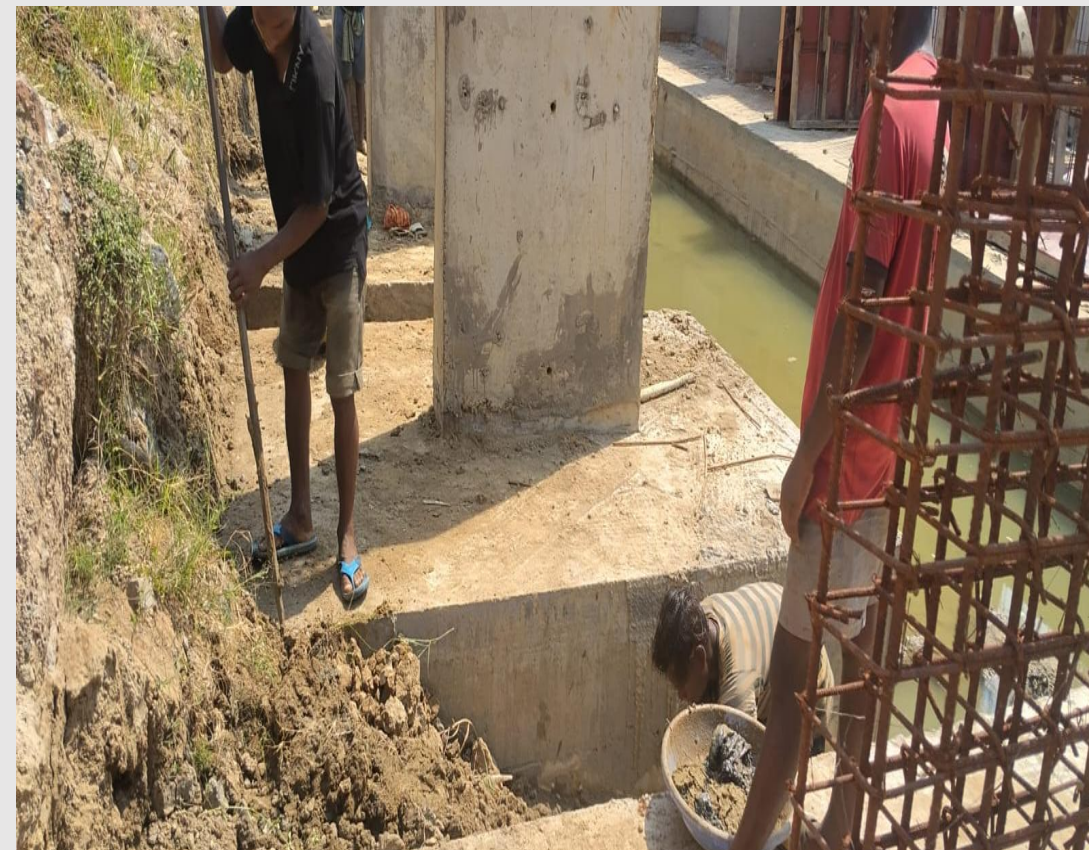
Slush Cleaning work in progress
