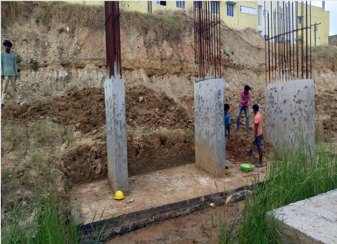
Slush Cleaning work in progress
