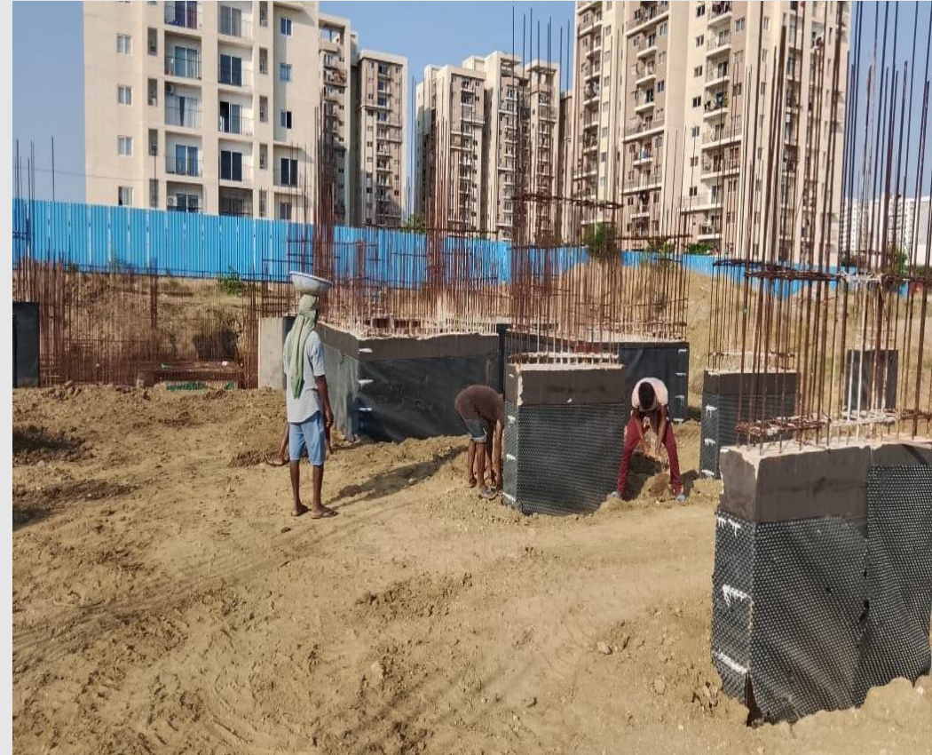
Roller compaction work in progress
