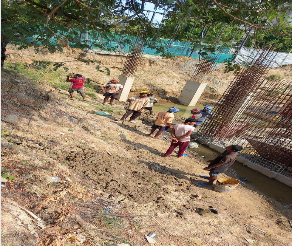
Tie Rod and Pipe removal in progress
