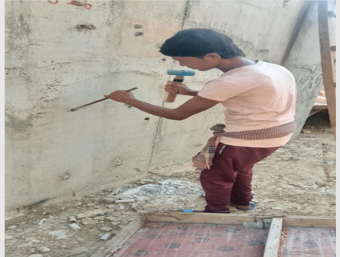
Tie Rod and Pipe removal work in progress
