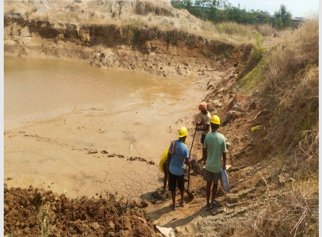
Slush removal work in progress
