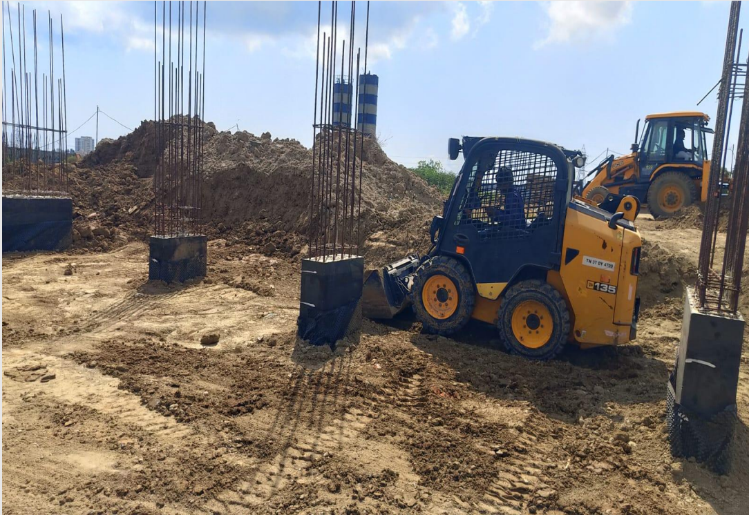
Earth filling work in progress
