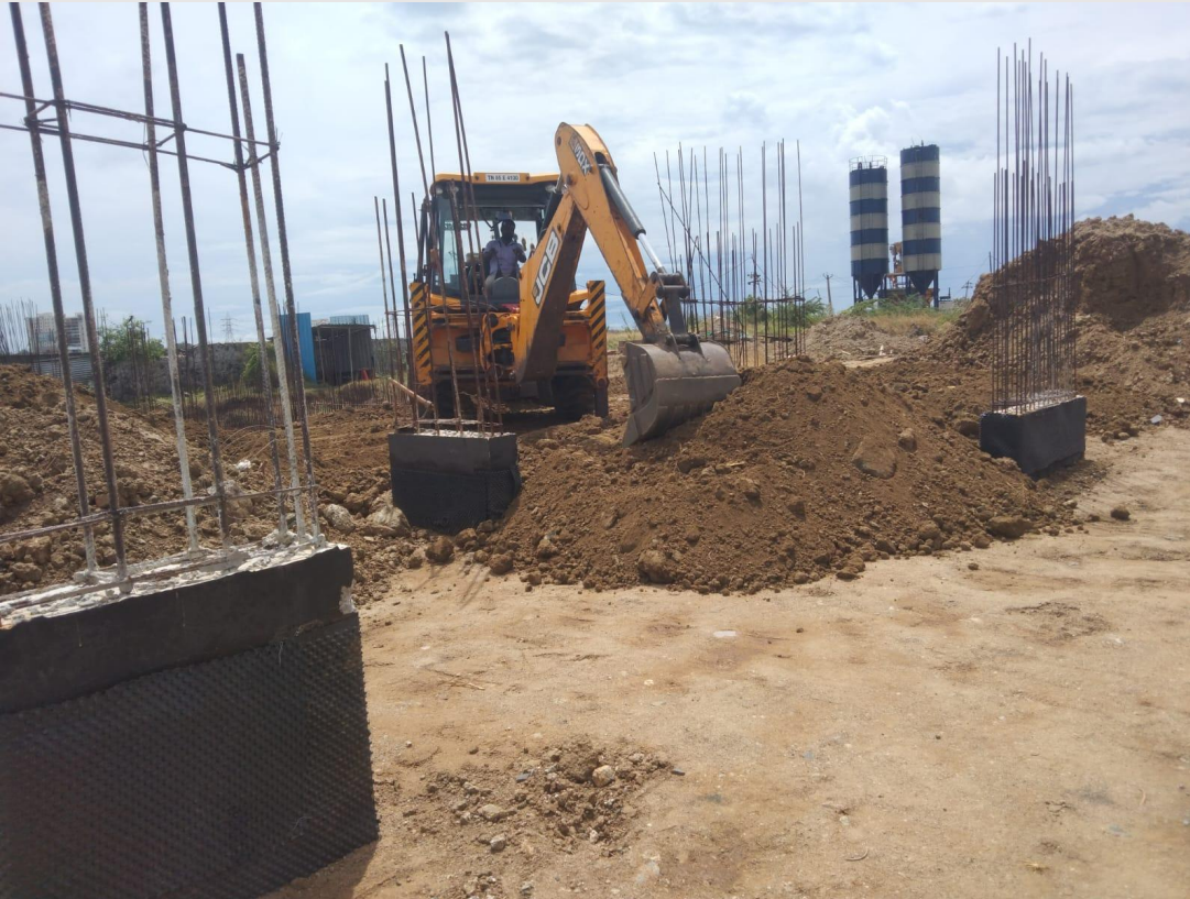
Soil Back filling work in progress
