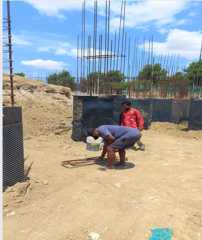
column reinforcement work
