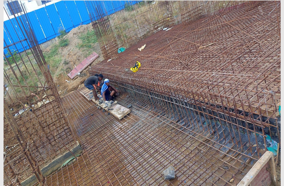
Raft brick work in progress
