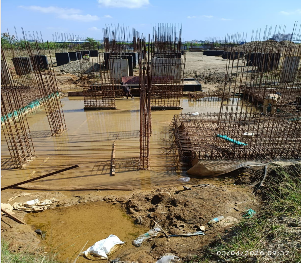
Raft cleaning work in progress
