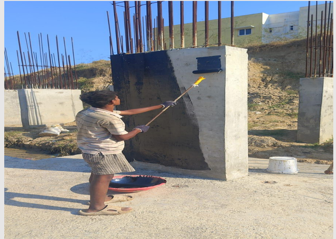
Water proofing and Epoxy coating work in progress
