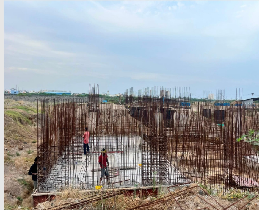
B5-UG Sump wall shuttering board making works and sump wall steel rust chemical coating works in progress
