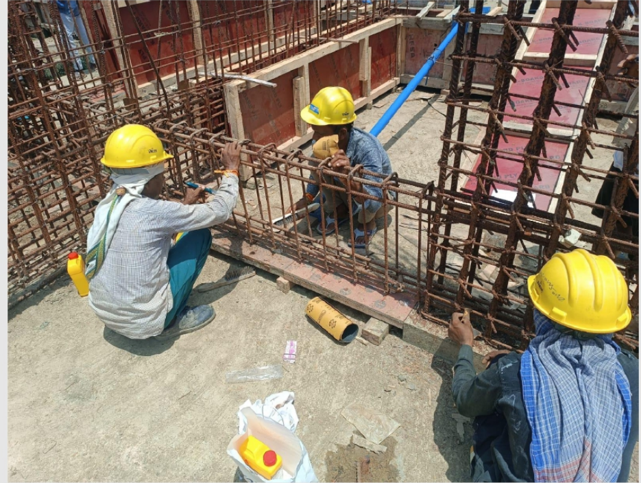
Reinforcement rust removal coating works in progress
