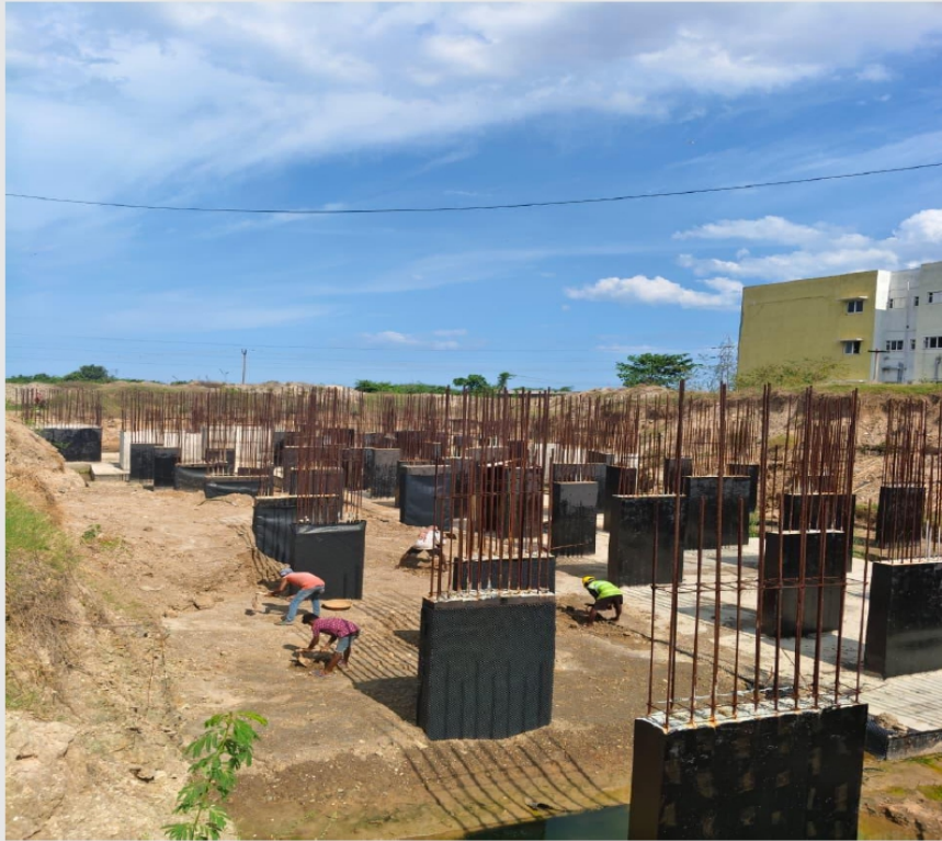
Soil levelling and compaction works in progress..
