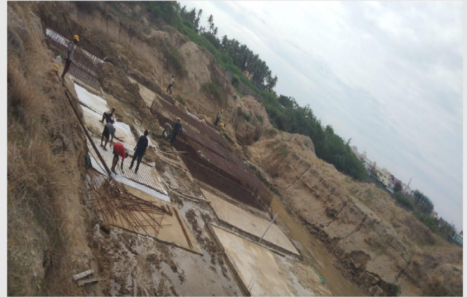
Footing reinforcement erection works in progress, sludge cleaning for PCC in progress.
