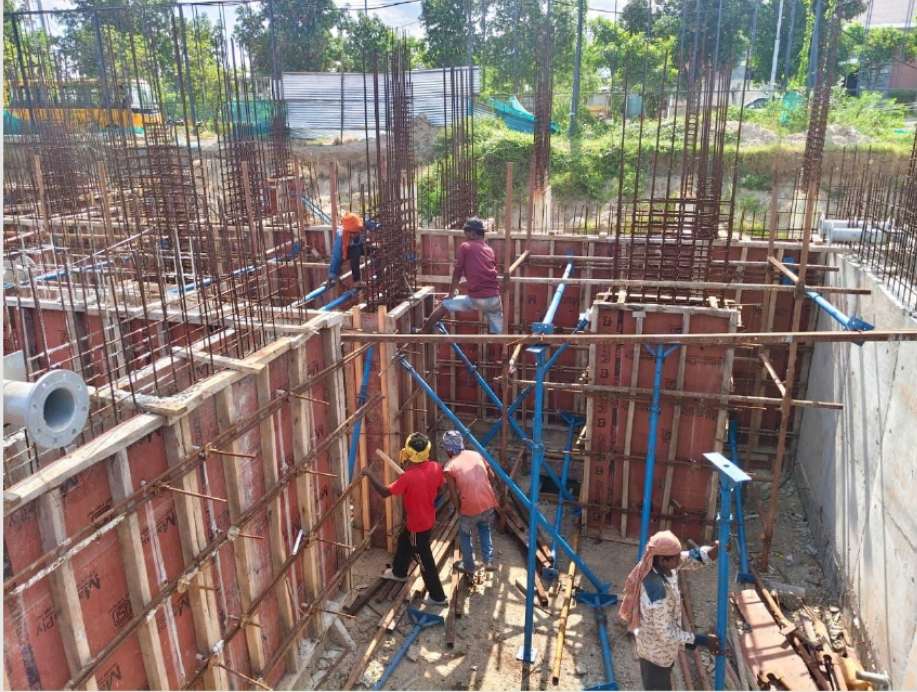
UG sump pump room and column shuttering supporting works in progress..
