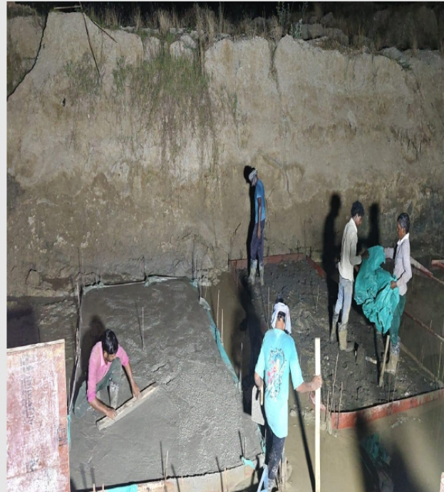
Footing PCC works in progress
