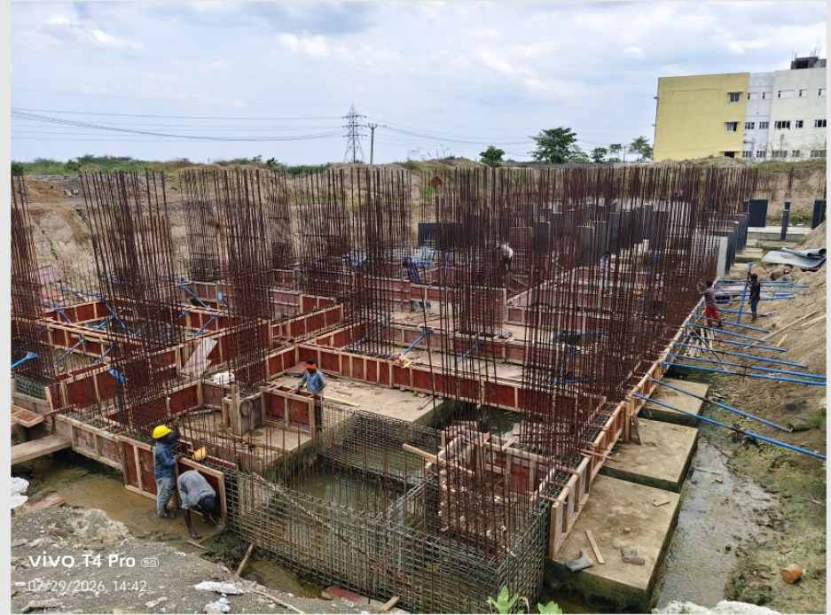
Sump plinth beam shuttering works
