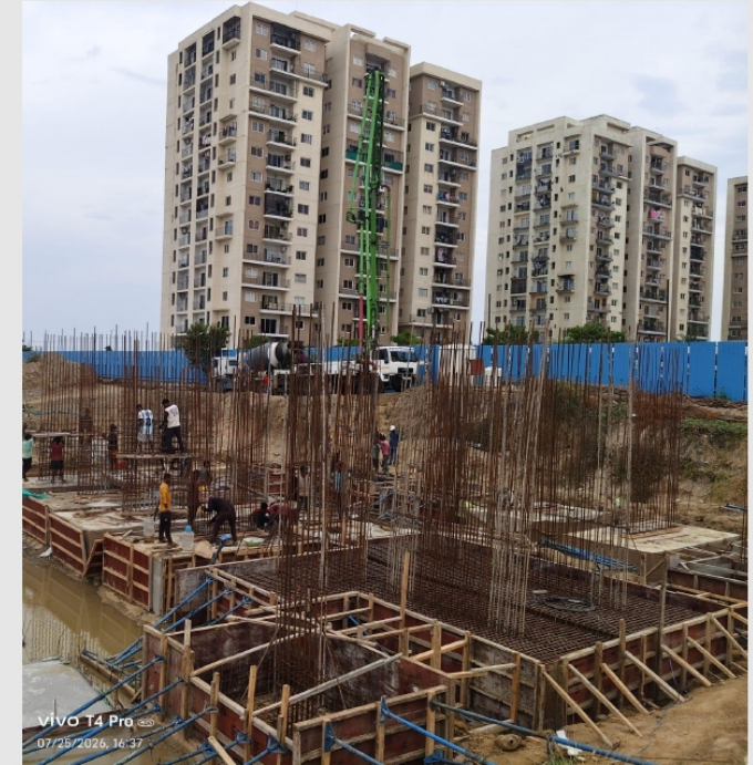
Footing concrete in progress
