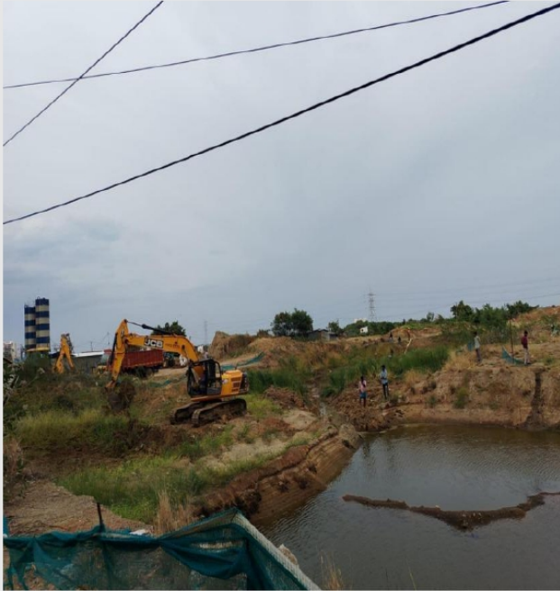
Excavation work commenced
