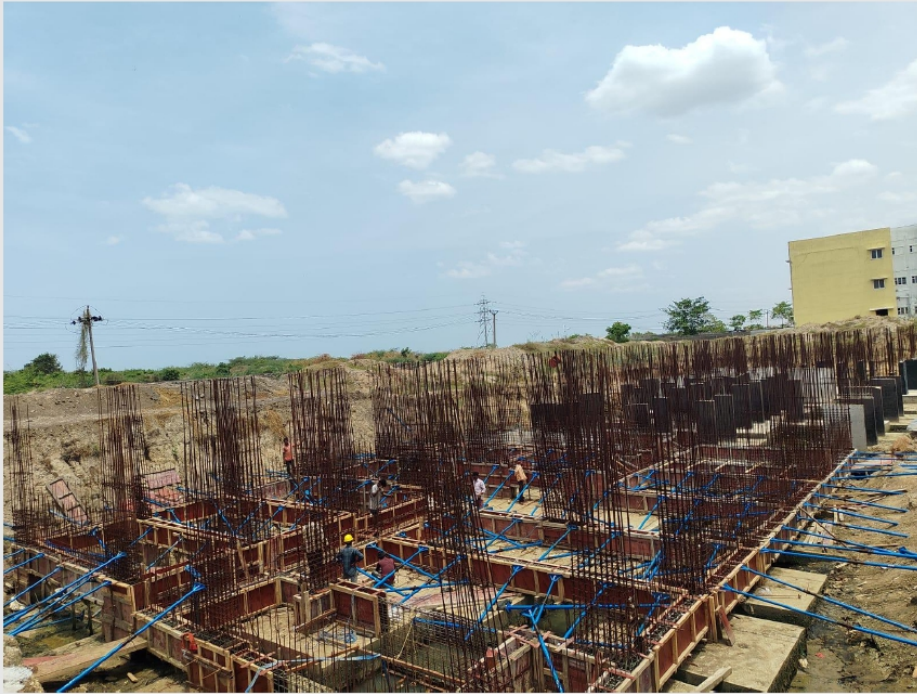
UG Sump plinth beam concrete planned
