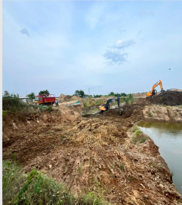
Excavation works in progress
