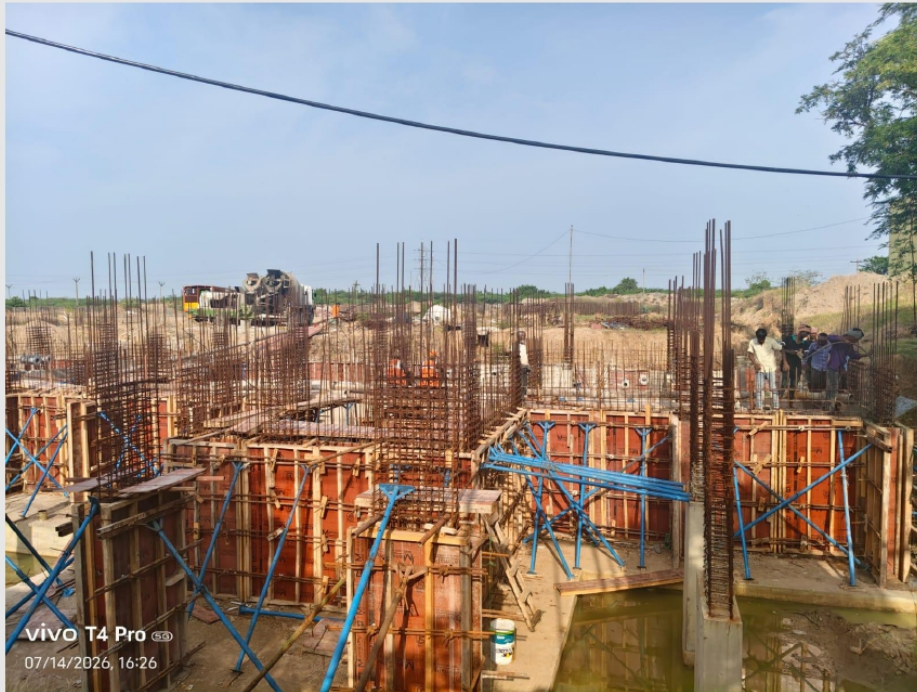
U G sump pump and 13 column concreting work in progress
