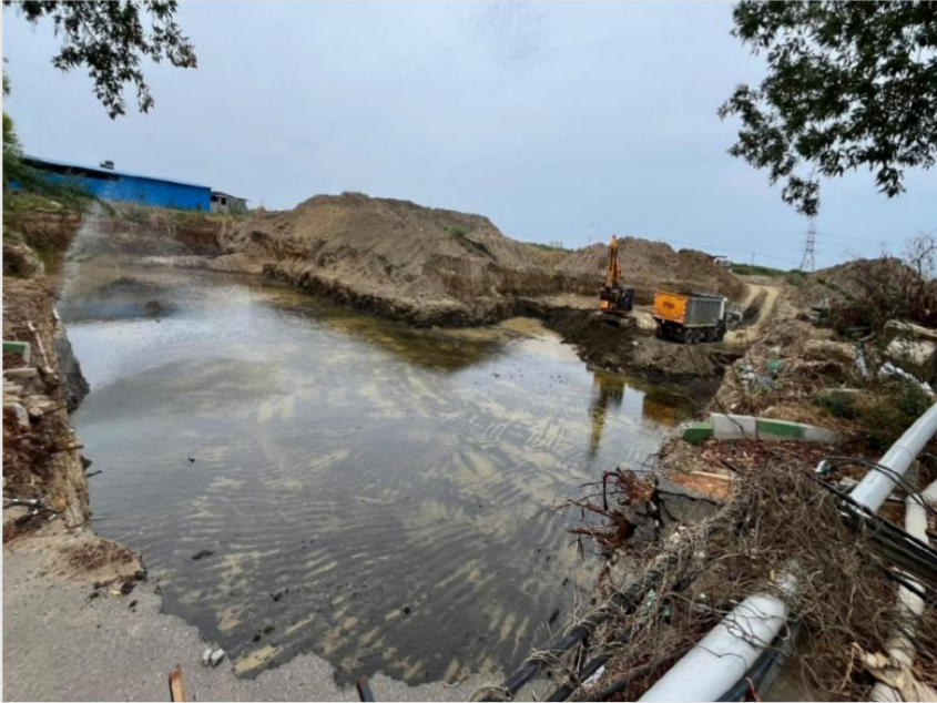
Excavation work in progress (Below 3M Depth)
