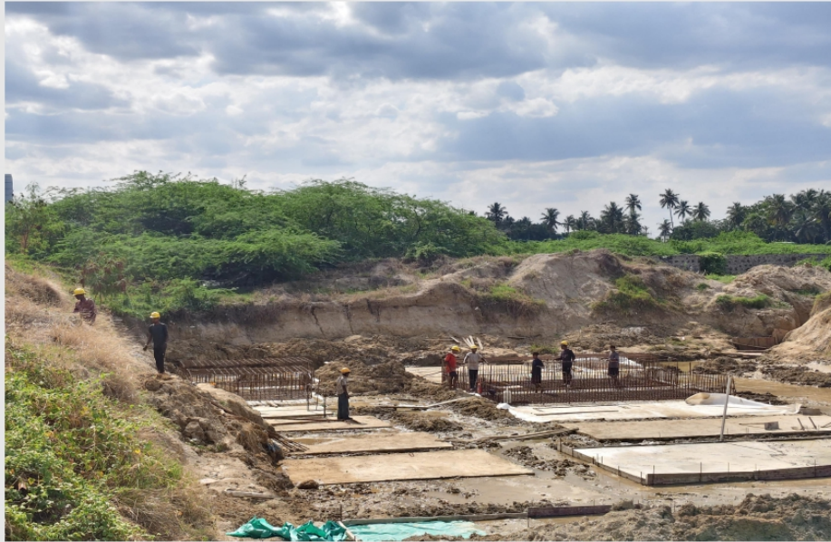
Footing reinforcement erection works in progress footing PCC Sludge removing work
