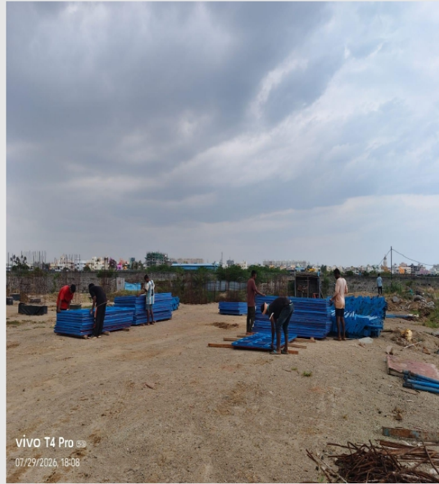
column and U G sump wall shuttering board making works in progress
