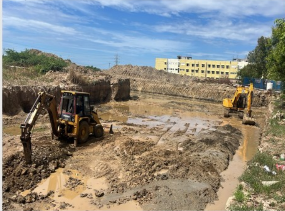
Excavation works in progress
