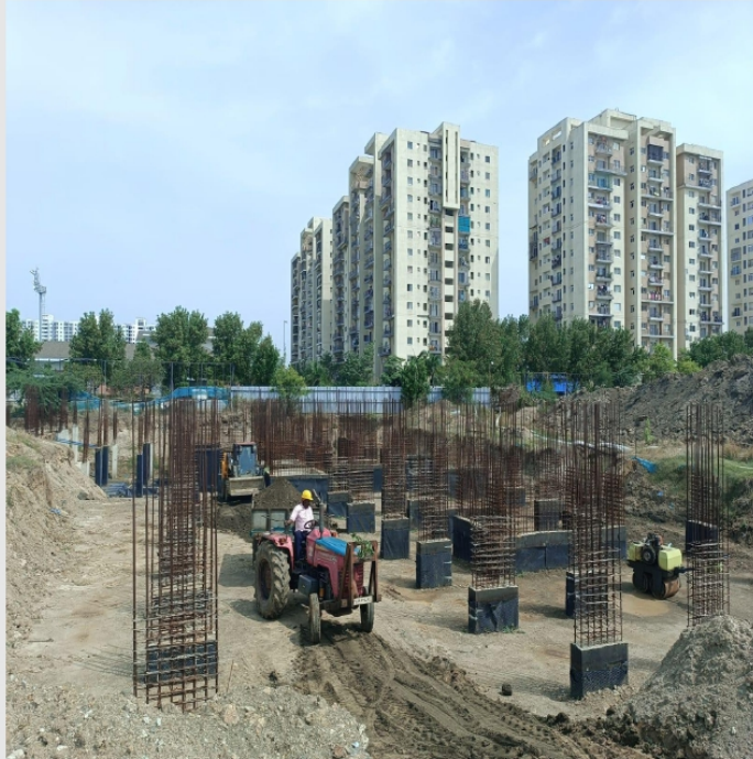
Curing works and deshuttering works in progress, north side final layer backfilling works in progress
