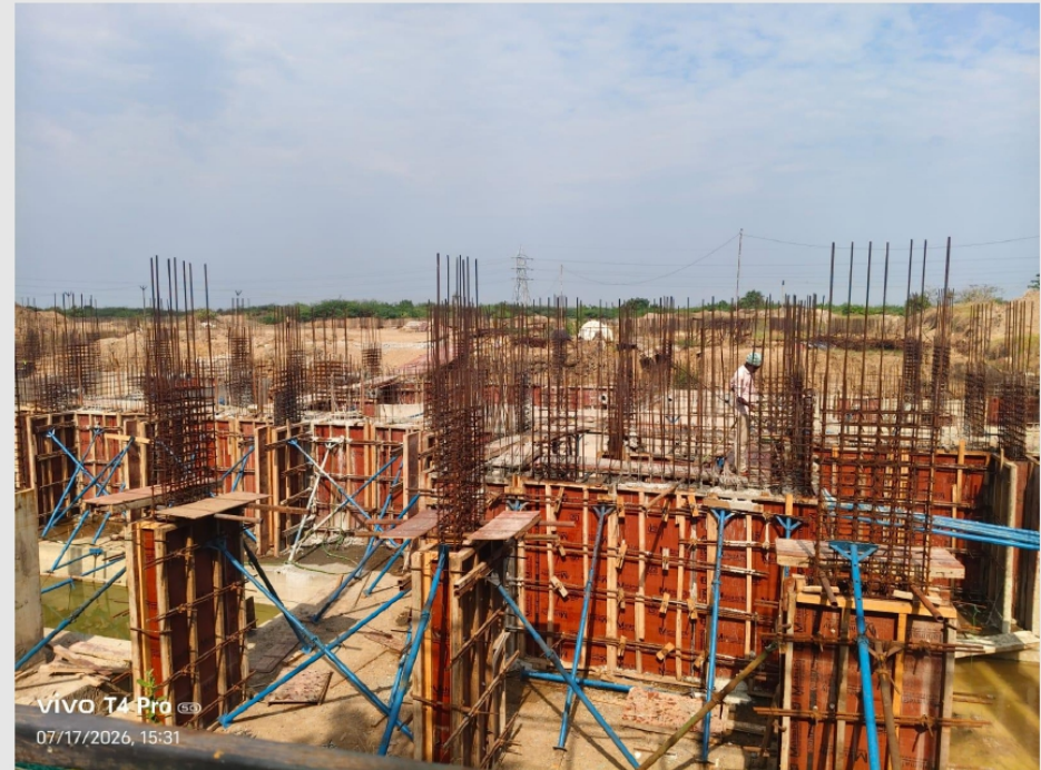
Concrete poured area curing works in progress
