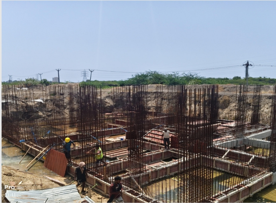
Plinth beam shuttering works in progress
