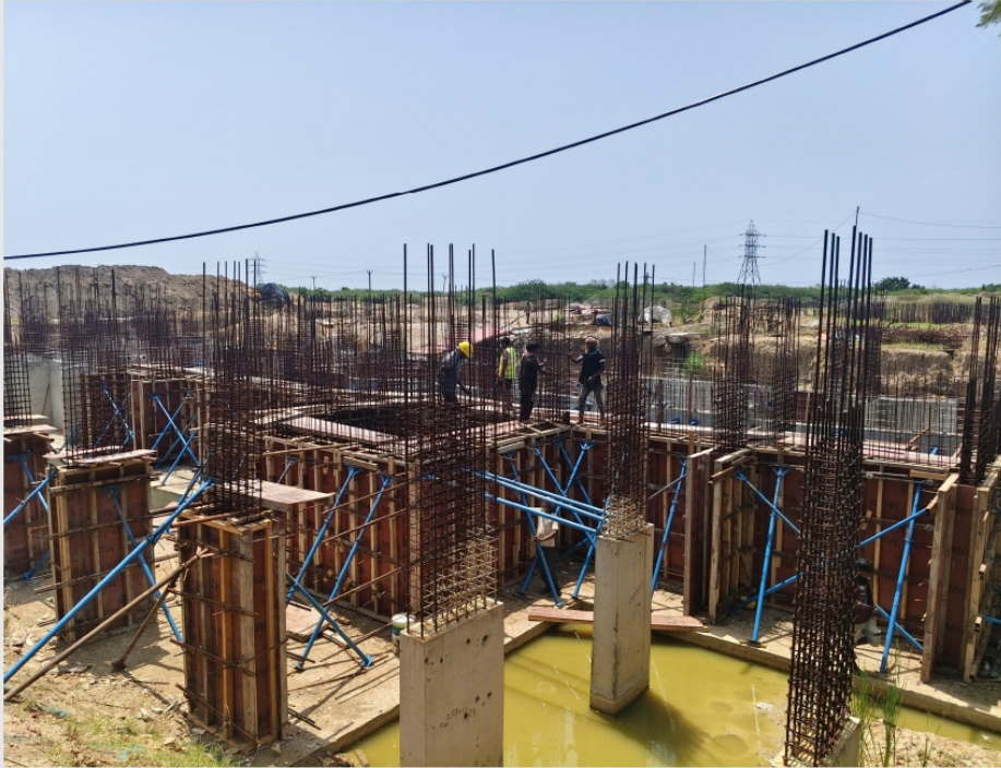
U G sump pump room and 13 column concrete planned
