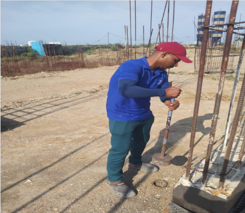
B5 & C1 soil compaction testing in progress
