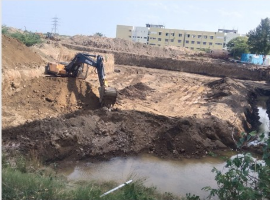
Excavation and rock strata chipping works in progress
