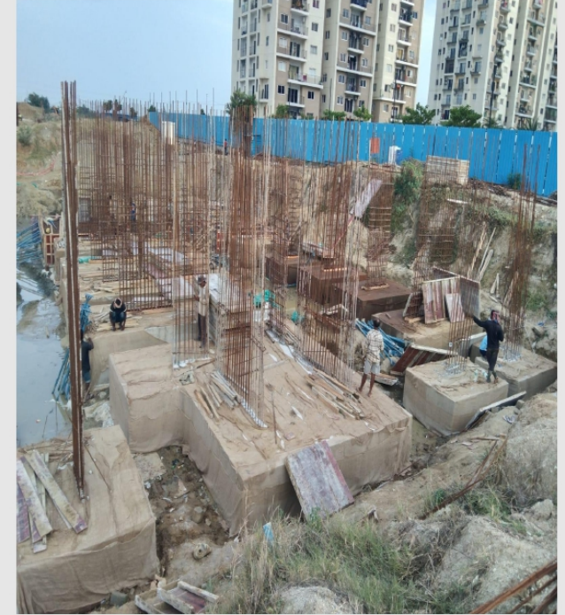
Footing reinforcement and shuttering works in progress footing PCC Sludge cleaning works in progress
