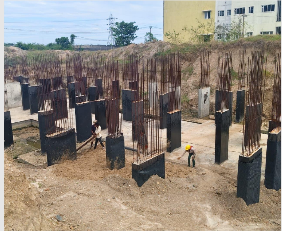
Soil levelling and compaction works in progress
