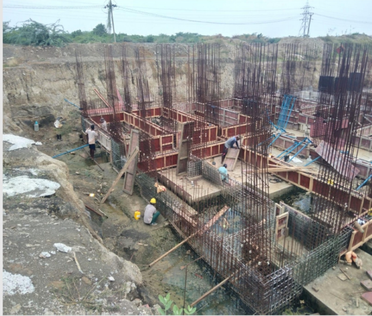
UG Sump plinth beam shuttering work is in progress
