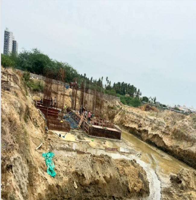
Footing and column reinforcement and footing shuttering works in progress. slush cleaning for PCC preparation
