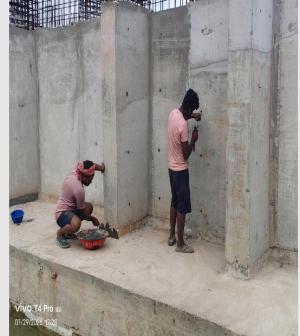
south side waterproofing coating preparation works
