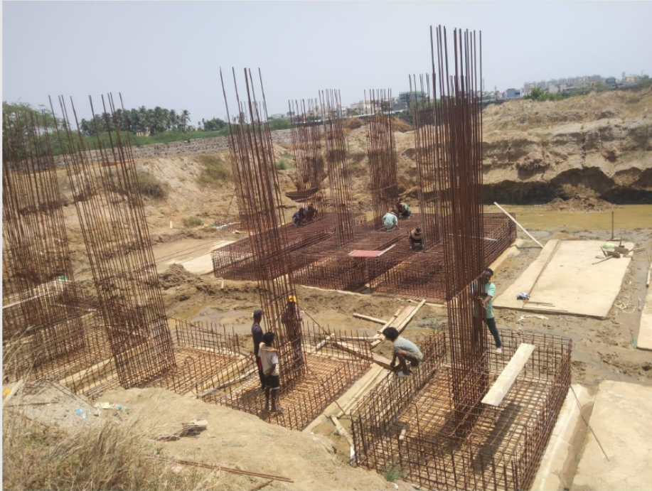
Footing and column reinforcement erection works in progress
