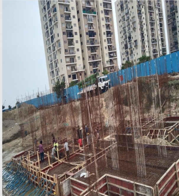
Footing and column reinforcement and footing shuttering works in progress. slush cleaning for PCC
