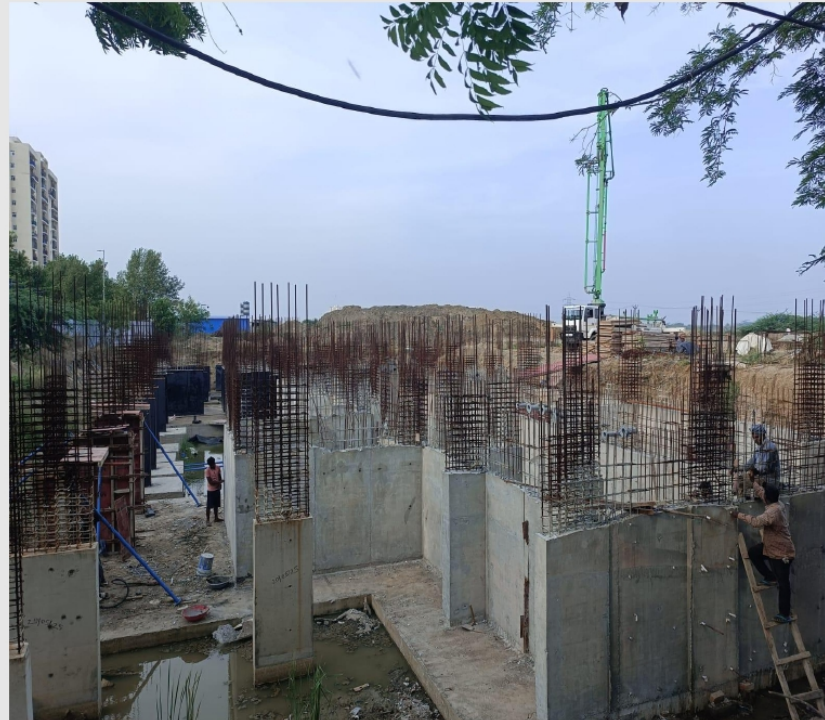
South side waterproofing coating preparation works in progress
