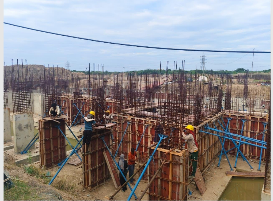
Column and shear wall shuttering supporting and alignment works in progress.
