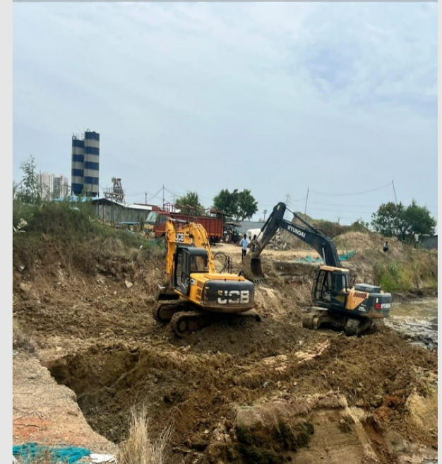
Excavation works in progress
