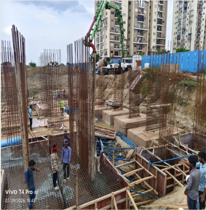
54Cum footing concrete in progress
