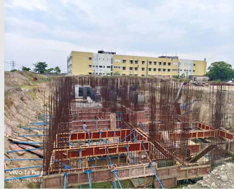
UG Sump plinth beam shuttering work is in progress. Waterproofing coating completed area protection sheet fixing works in progress
