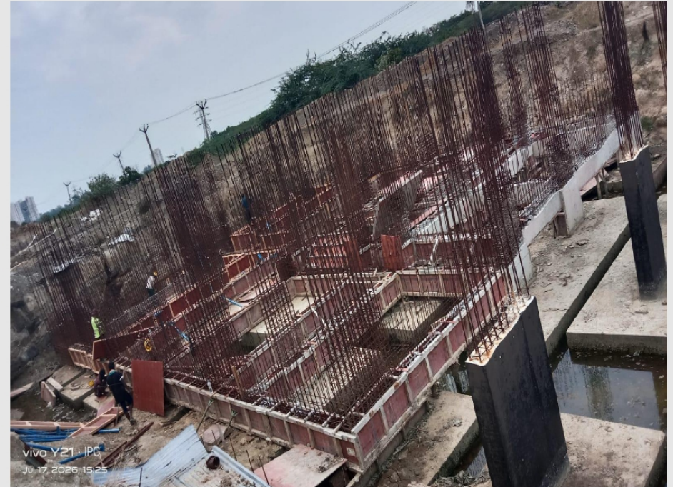
U G sump plinth beam shuttering works in progress
