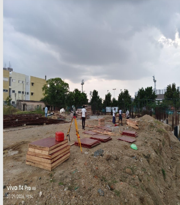
2nd lift column shuttering board making works in progress
