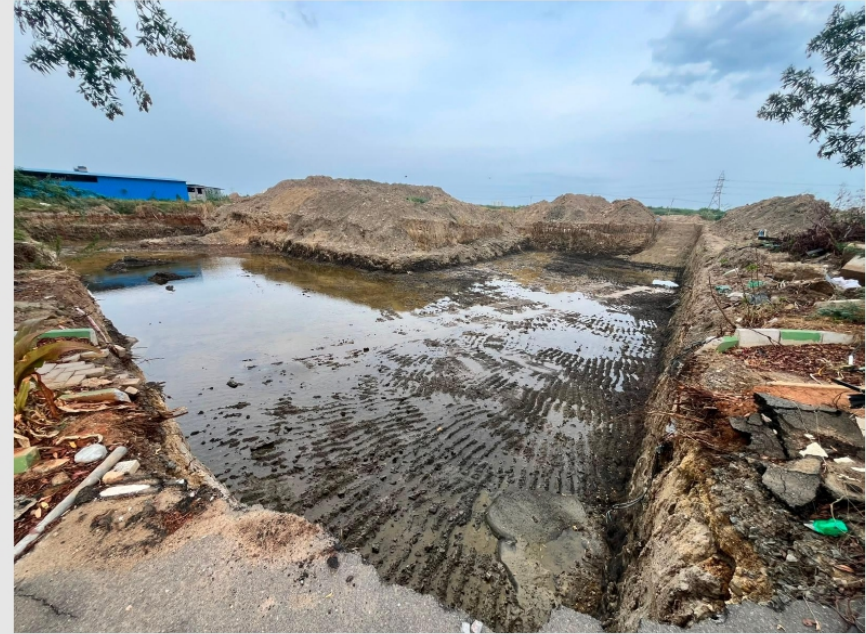
Excavation work completed upto 4m depth, awaiting for consultant formation
