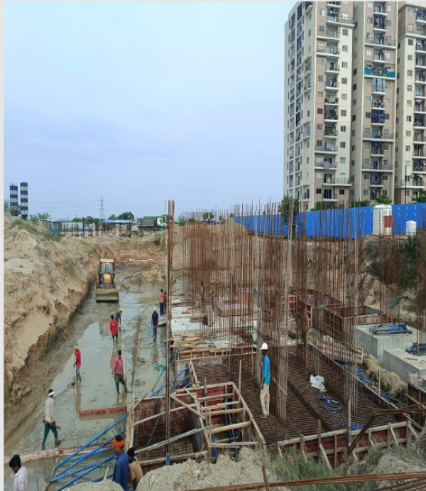
Footing PCC concrete 7cum planned today Footing RCC 90cum planned
