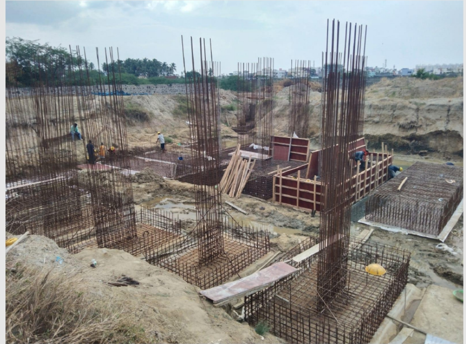
Footing & Column reinforcement and shuttering works in progress, Sludge cleaning for footing PCC works in progress
