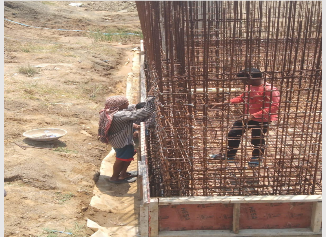
UG Sump shuttering work in progress.
