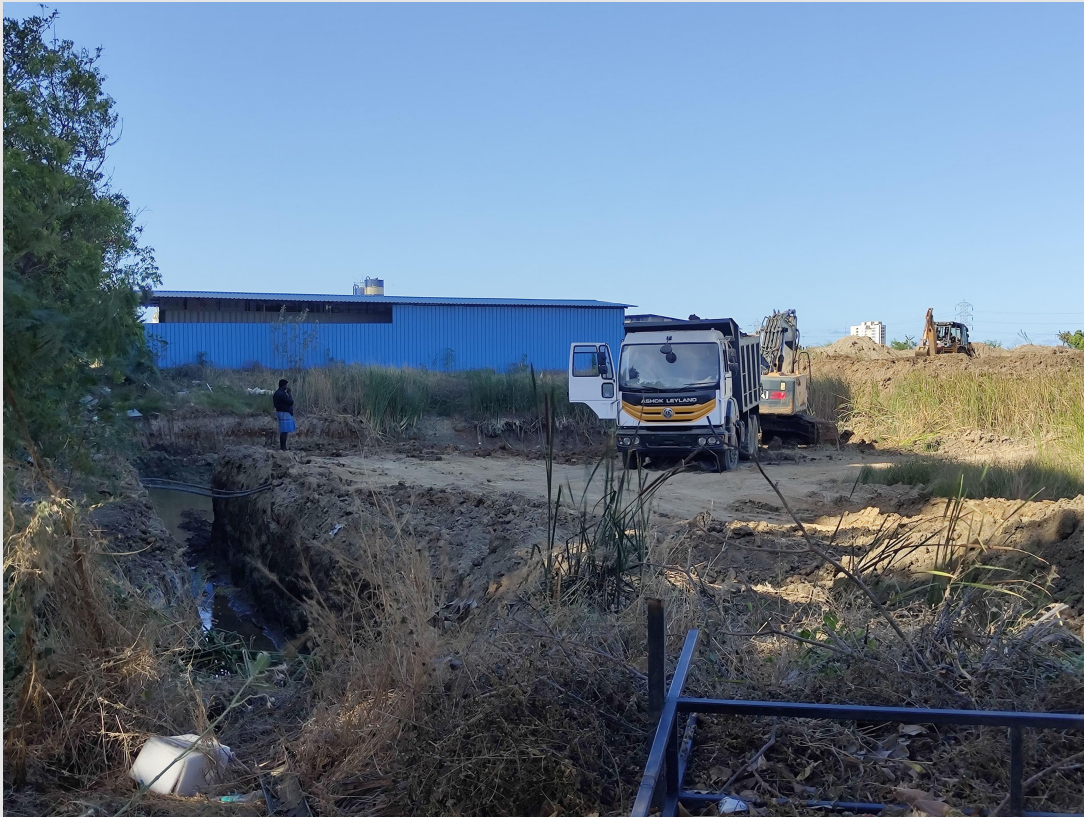
Excavation work in progress
