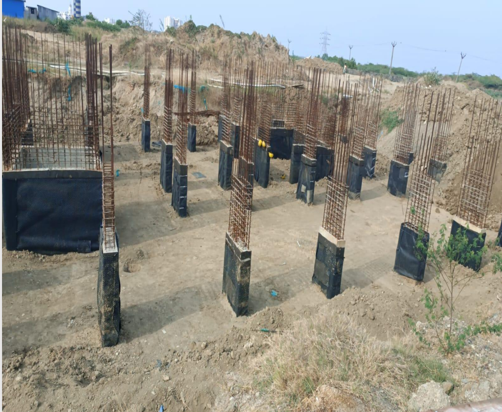
Soil compaction work in progress
