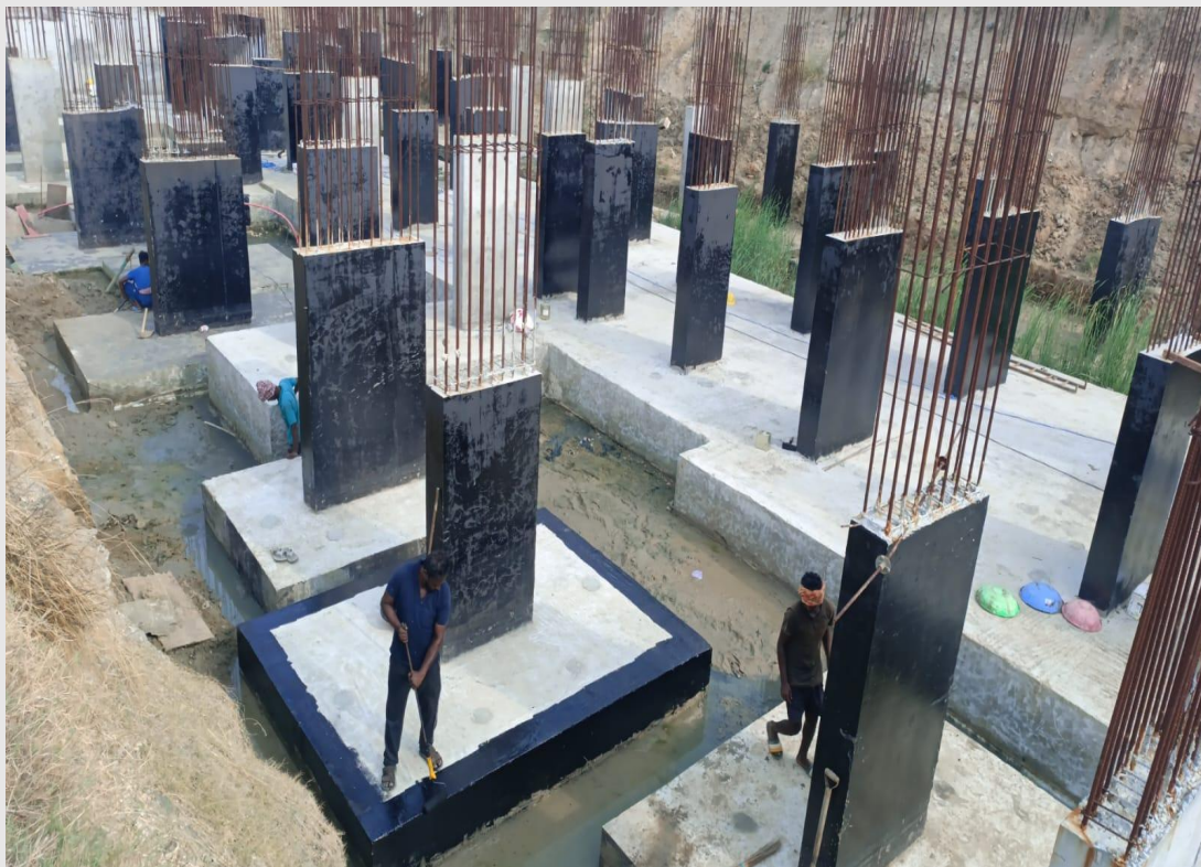
Waterproof coating work in progress
