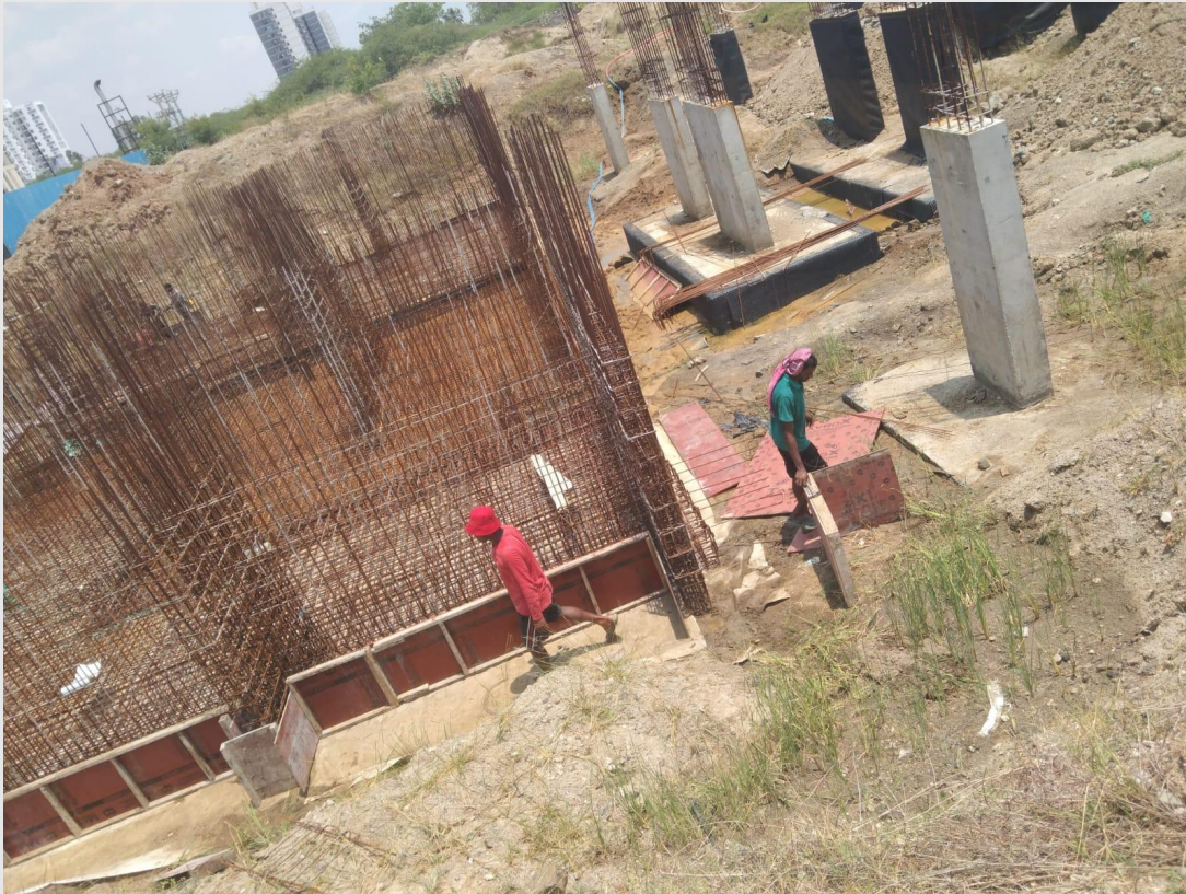
UG Sump shuttering in progress
