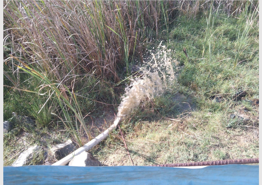
Dewatering in progress
