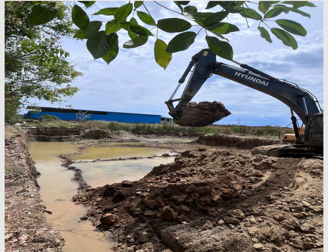
Excavation along with dewatering work in progress
